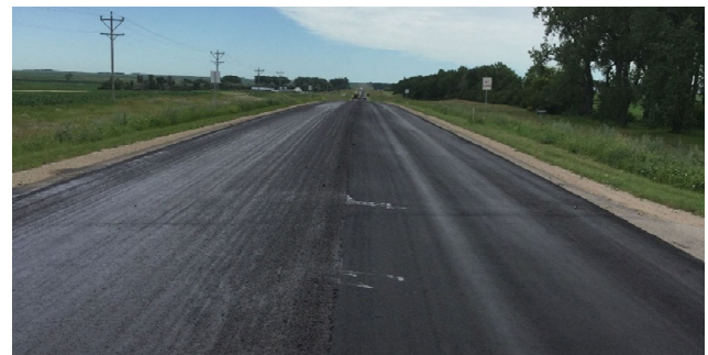
RAP Slurry Seal
