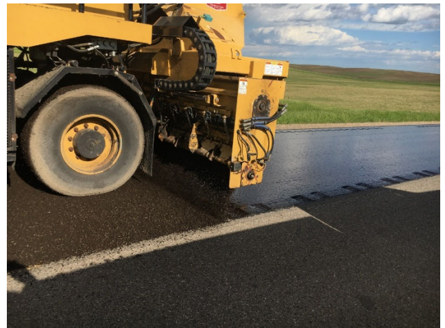
Placing the RAP Chips
