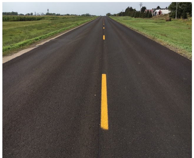
Finished and ready for new rumble strips
