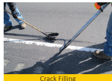
Crack Sealing
