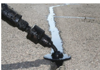
Routed crack being sealed
