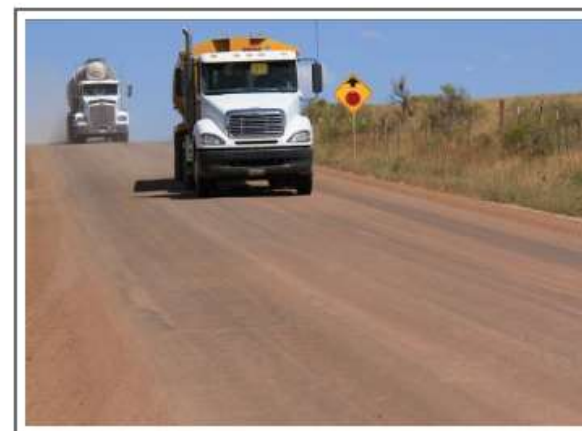
Stable fines preservation on a treated road
