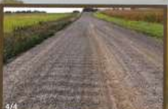
4/4 POOR: 10-7-13 After another 0.3 gal per sq yd was applied same season still not performing well. This is such poor surface material it won't go into a bound state no matter how you maintain it. There is no way the MgCl_2 can work even with 0.8 gal per sq yd applied in one year!
