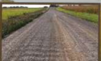
4/4 POOR: 10-7-13 After another 0.3 gal per sq yd was applied same season still not performing well. This is such poor surface material it won't go into a bound state no matter how you maintain it. There is no way the MgCl_2 can work even with 0.8 gal per sq yd applied in one year!
