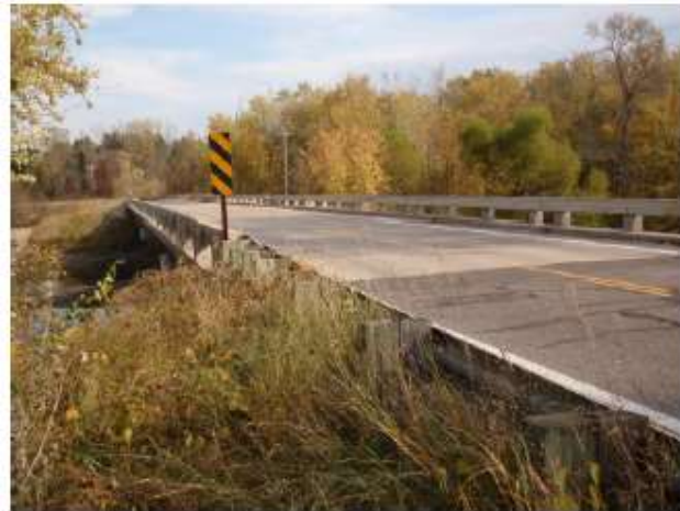
1. Roadway across Bridge
