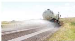
Spreading Slurry
