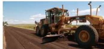
Blade Mixing Slurry
