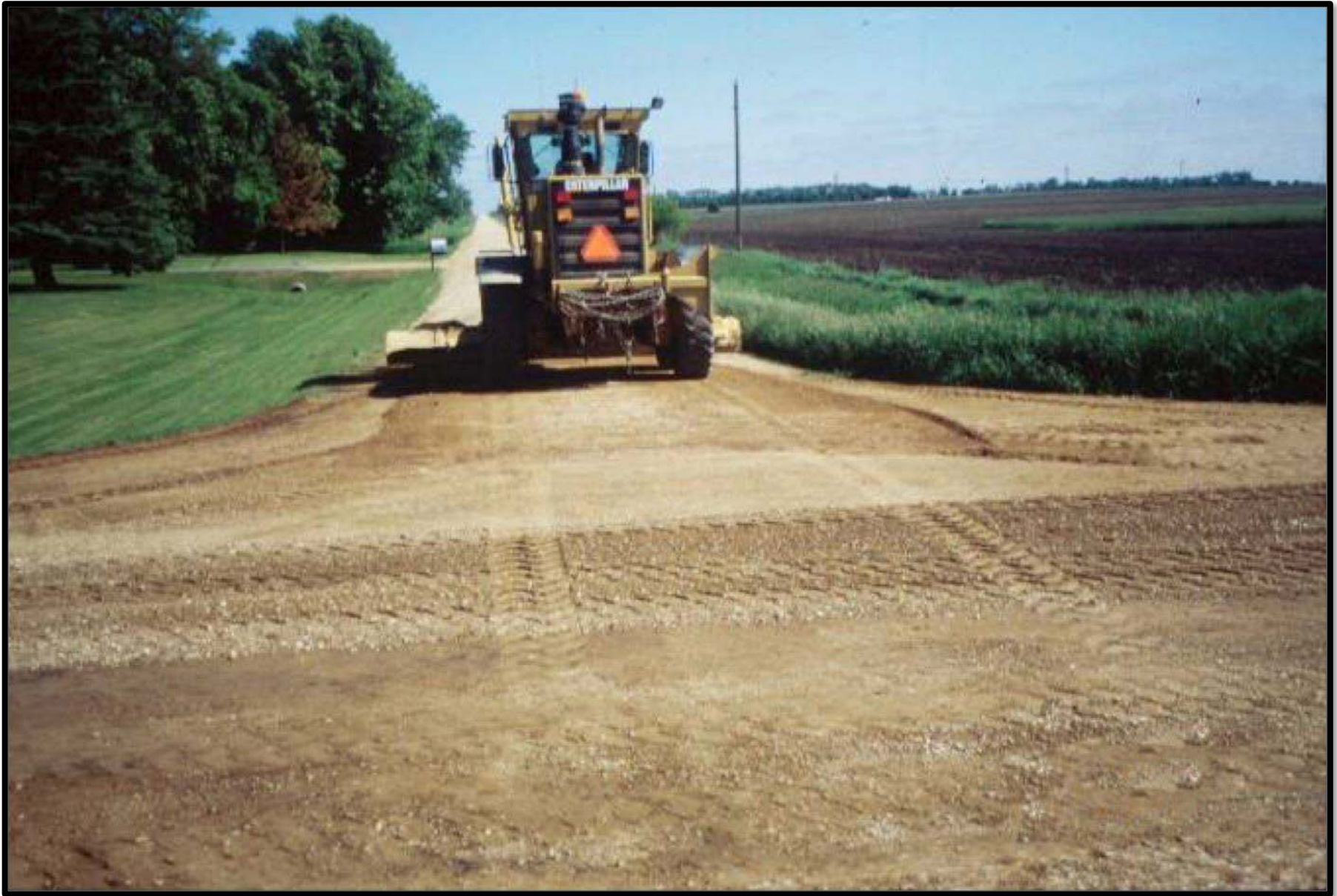
Flattening the immediate approach to the intersection to match.
