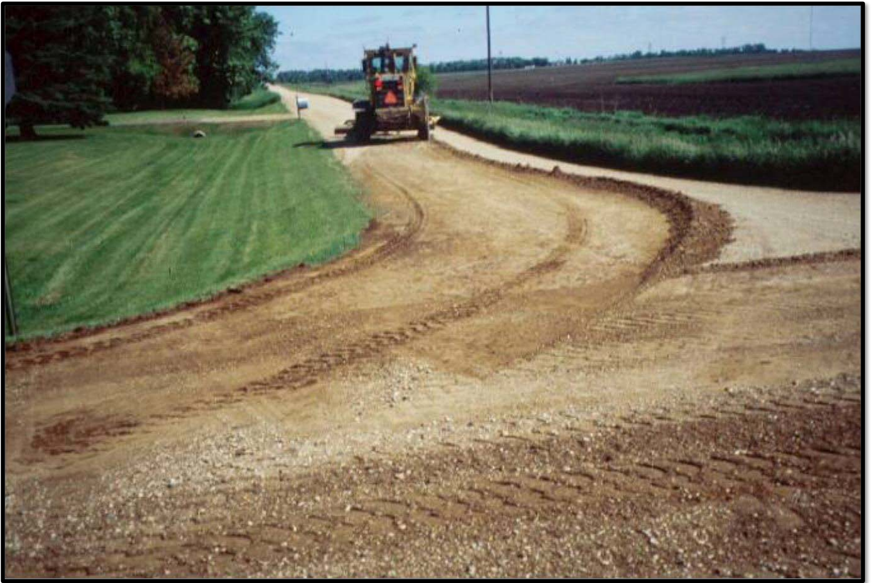
Shaping the corner leaving the material to work the crown
