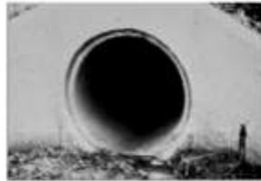
Headwall - Groove Edge (applies to Concrete pipe with the socket end in combination with a concrete headwall)
