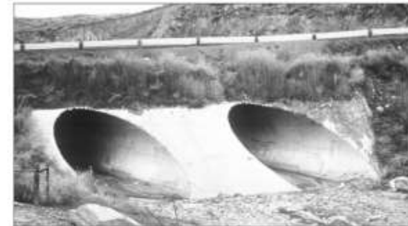
Miter/Square/2:1 Slope (applies to CMP, PVC plastic, Smooth HDPE or Corrugated PE culverts that are mitered to conform to the slope)
