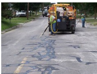
Crack sealing in the field
