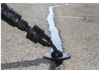
Routed crack being sealed
