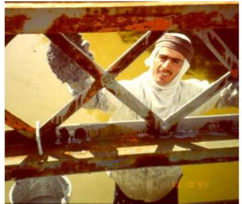
Figure 30. Coating application on riveted steel using a mitt
