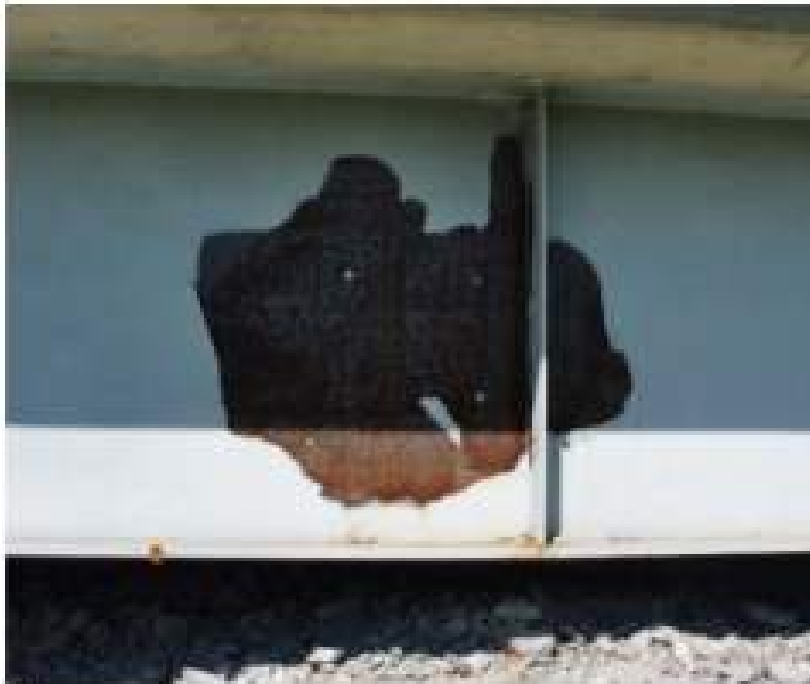
Coating Failure Exposing Rusty Mill Scale
