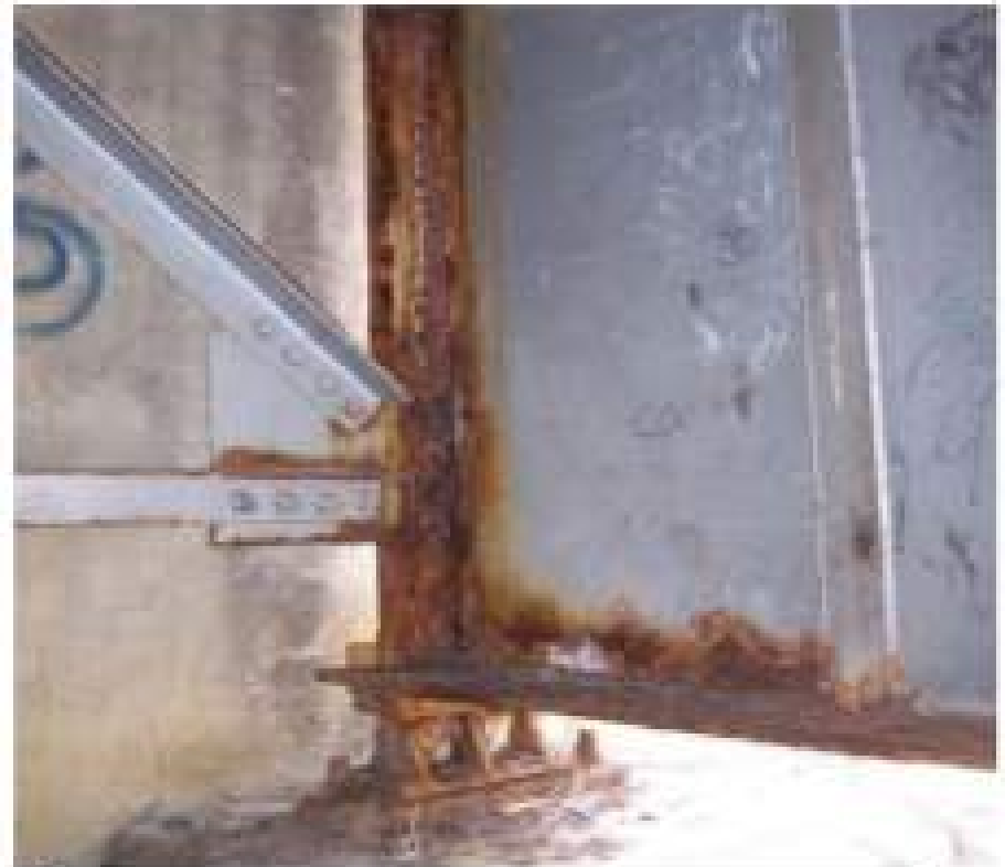
Corrosion of Beam End, Cross Frame and Bearing
