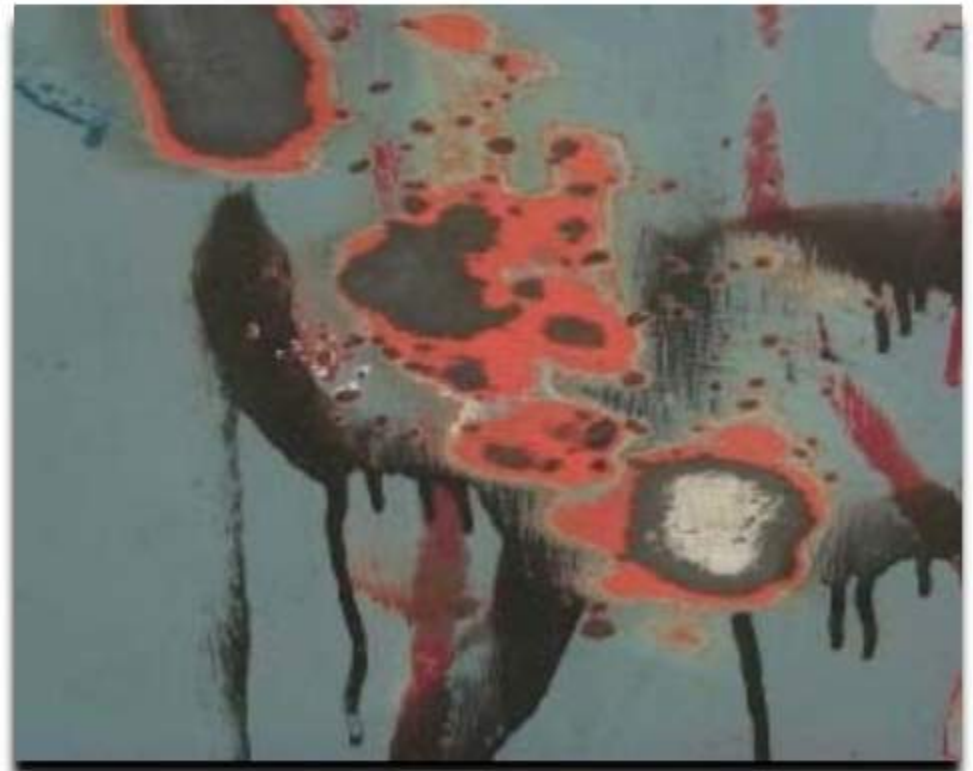
Figure 25. Feathering of existing coating
