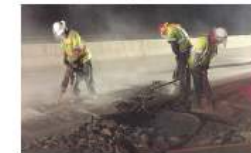
DETERIORATED DECK CONCRETE REMOVAL
