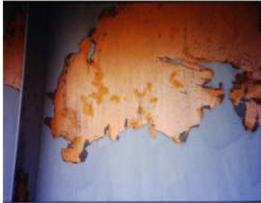
Inter-Coat Failure
