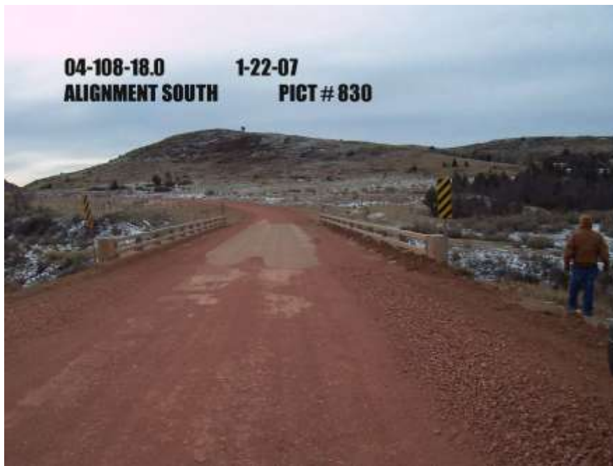
ADT = 50-100 Well graded and maintained, good gravel or paved surface, tracks indicate that 2 vehicle operation is normal
