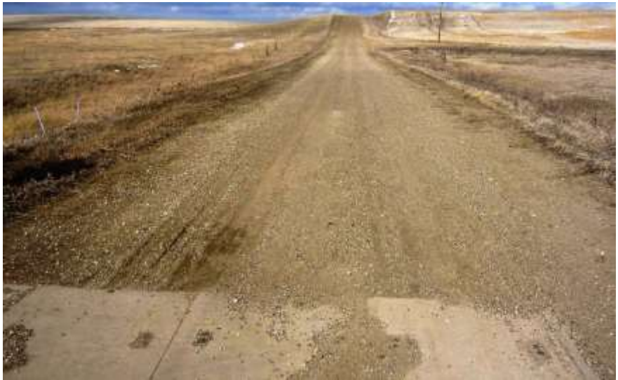
ADT = 20 Two tracks, grade raise apparent, gravel surface, continual single vehicle use
