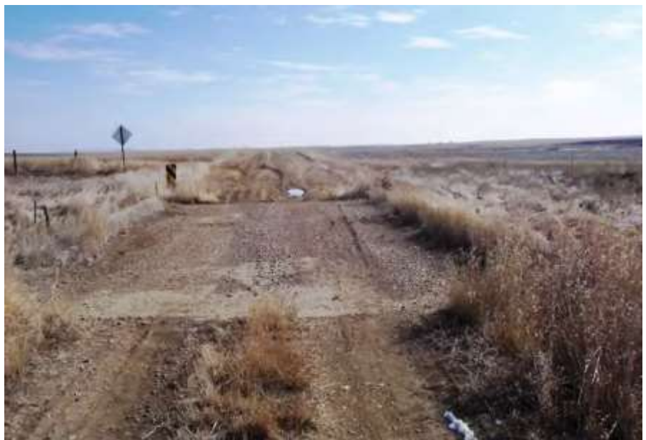
ADT = 10 Two tracks, no appreciable grade raise, some continual use apparent
