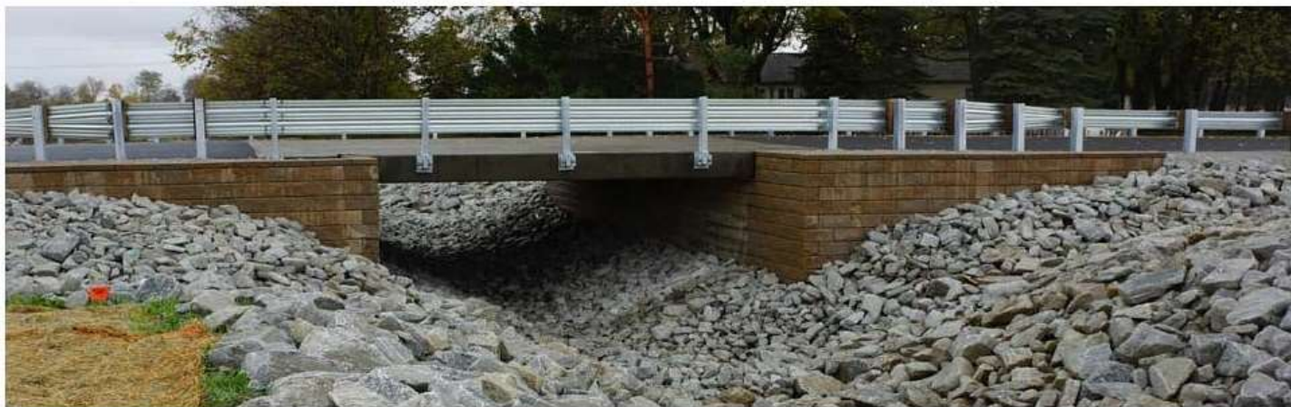
This is an example of an accelerated bridge construction utilizing permanent steel sheet piles supplied by Skyline
