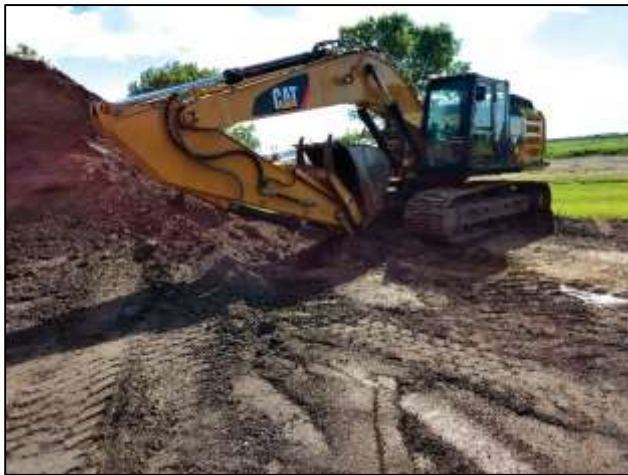
Figure 3. Backhoe for Removing RAP
