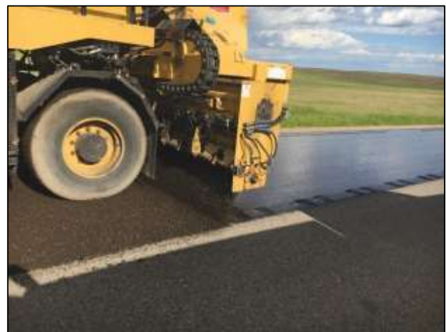
Figure 9. Application of RAP Chip Seal
