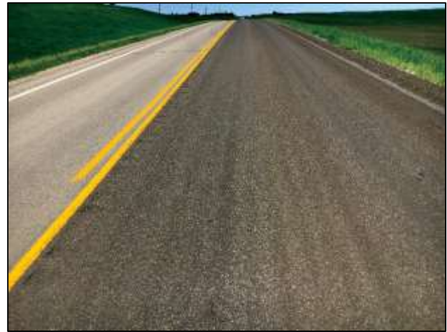
Figure 8. Test Section 1 – Right Lane
