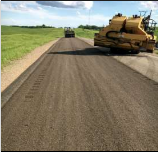
Figure 11. RAP Chip Seal after Application
