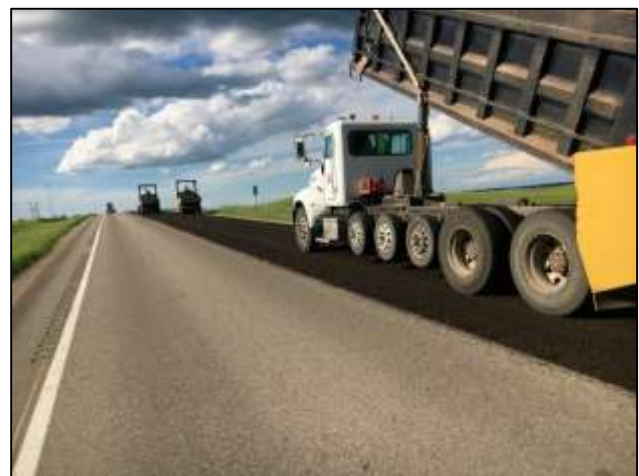
Figure 10. Application of RAP Chip Seal
