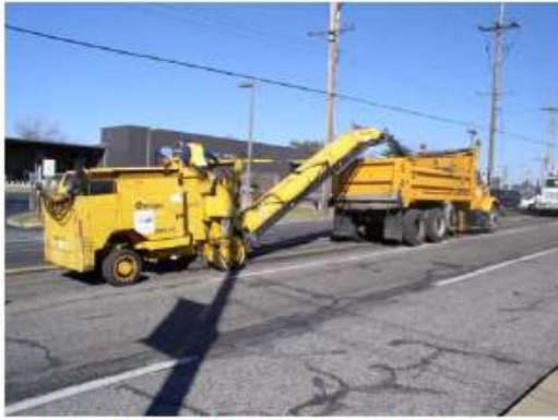
(1) Pavt Repair Milling Operation
