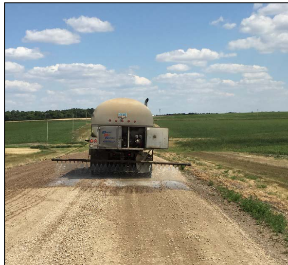
Calcium Chloride dust suppressant helps consolidate the road surface and provides a dust-free driving surface and environment.
