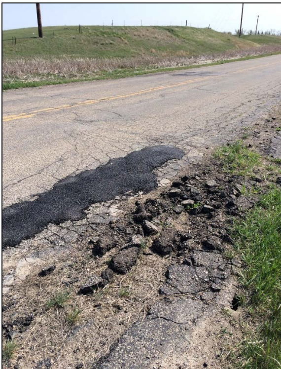
State Highway 2 before conversion
