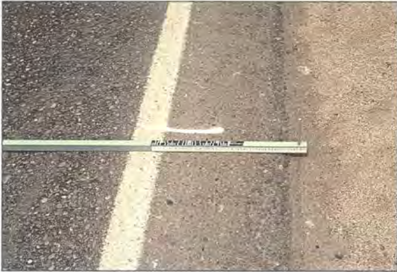
Figure 44: Distress Type ACP 14 Lane-to-Shoulder Dropoff
