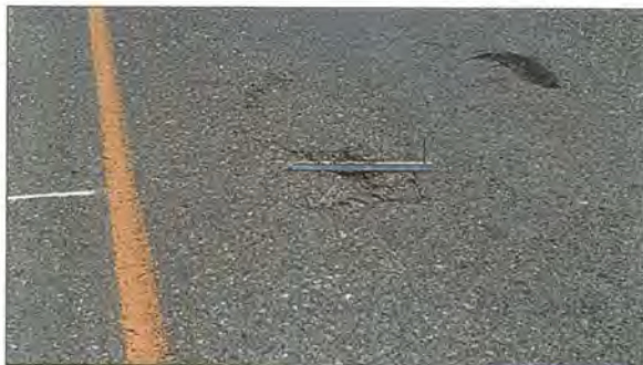
Figure 27: Distress Type ACP 8 Low Severity Pothole
