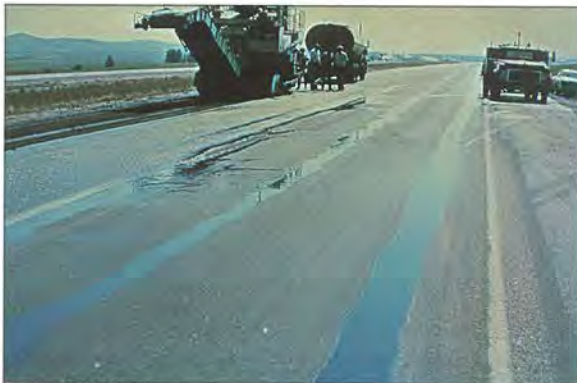
Figure 33: Distress Type ACP 9 Standing Water in Ruts
