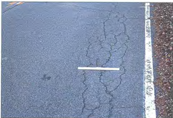
Figure 6: Distress Type ACP 1 Moderate Severity Fatigue Cracking
