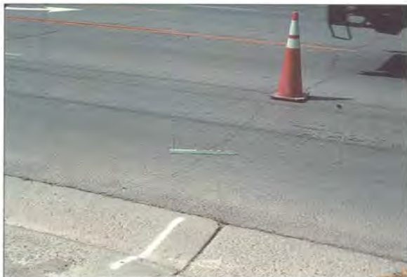
Figure 20: Distress Type ACP 6 Moderate Severity Transverse Cracking
