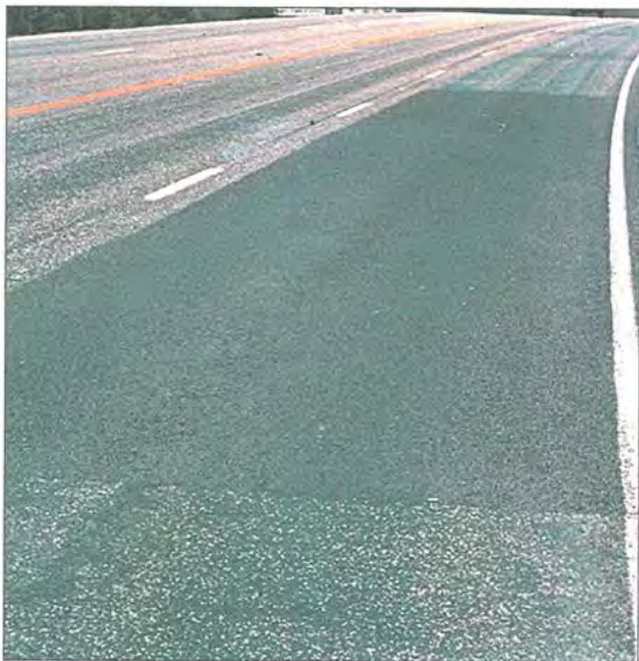
Figure 23: Distress Type ACP 7 Low Severity Patch
