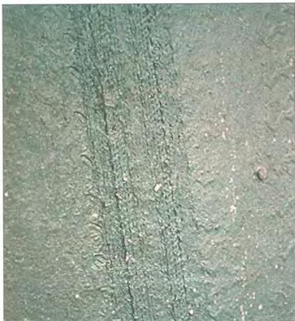
Figure 38: Distress Type ACP 11 High Severity - Aggregate Obscured
