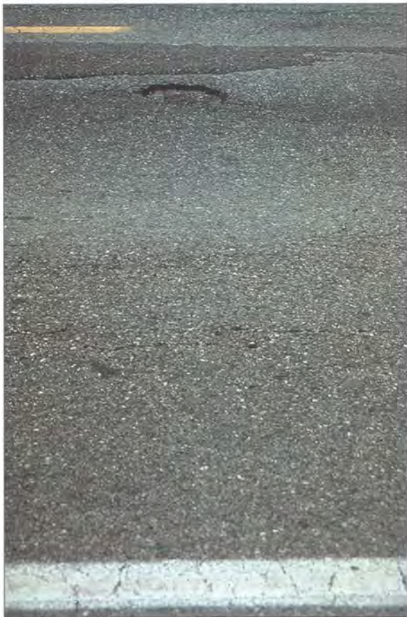
Figure 28: Distress Type ACP 8 Moderate Severity Pothole
