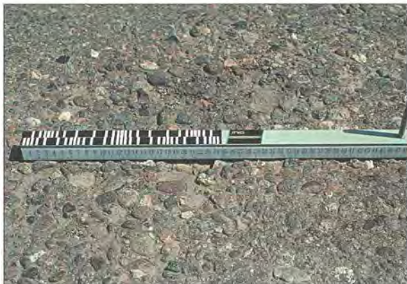
Figure 42: Distress Type ACP 13 Loss of Coarse Aggregate
