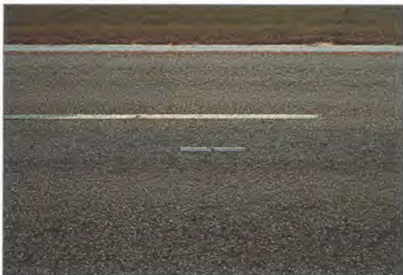
Figure 36: Distress Type ACP 11 Low Severity - Discoloration
