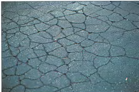
Figure 4: Distress Type ACP 1 Chicken Wire/Alligator Pattern Cracking Typical in Fatigue Cracking
