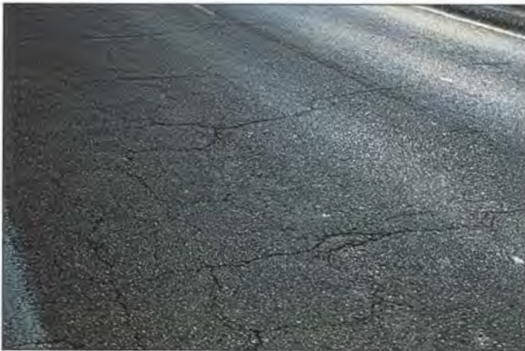
Figure 10: Distress Type ACP 2 High Severity Block Cracking
