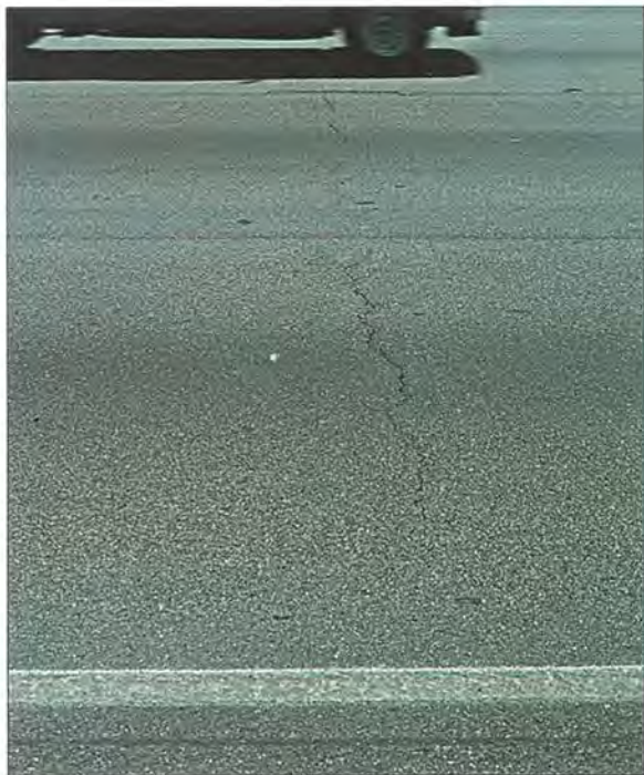
Figure 19: Distress Type ACP 6 Low Severity Transverse Cracking
