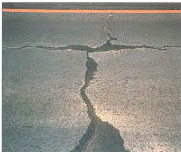
Figure 45: Distress Type ACP 15 Water Bleeding and Pumping
