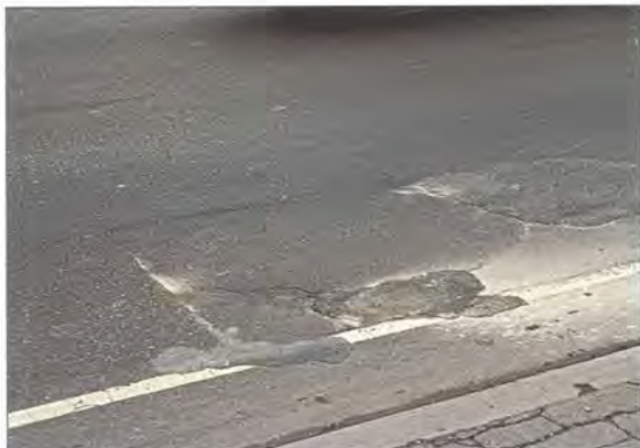
Figure 25: Distress Type ACP 7 High Severity Patch
