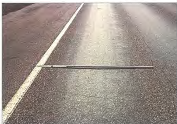
Figure 32: Distress Type ACP 9 - Rutting
