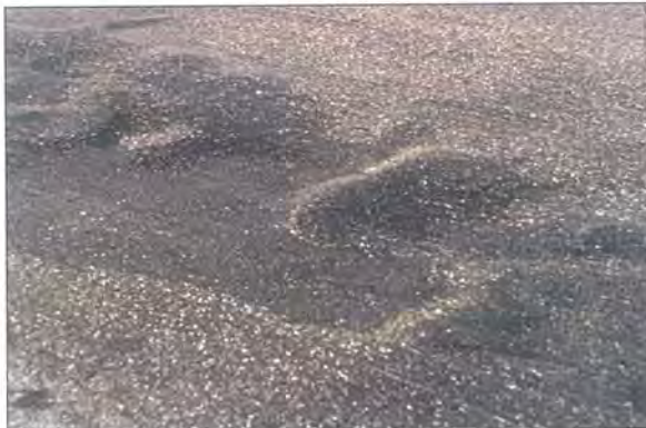
Figure 35: Distress Type ACP 10 Shoving in Pavement Surface
