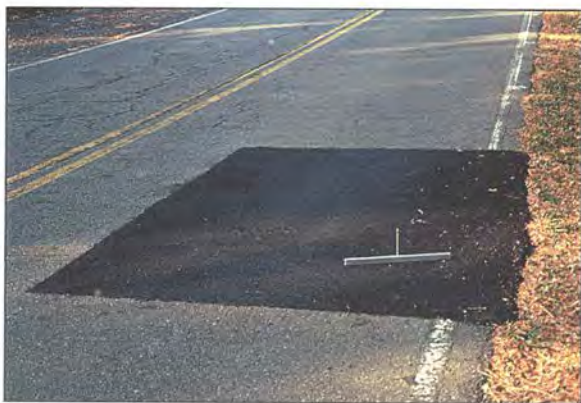
Figure 24: Distress Type ACP 7 Moderate Severity Patch
