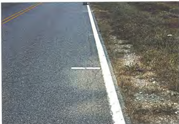
Figure 12: Distress Type ACP 3 Low Severity Edge Cracking
