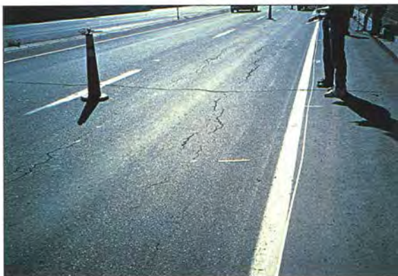
Figure 5: Distress Type ACP 1 - Low Severity Fatigue Cracking
