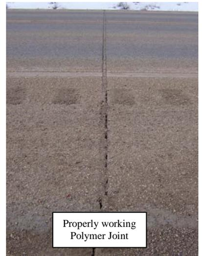
Properly working Polymer Joint
