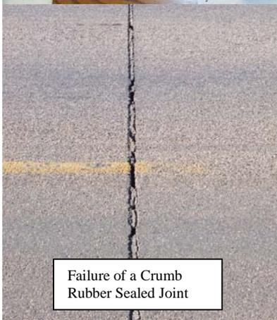
Failure of a Crumb Rubber Sealed Joint
