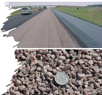
Asphalt Surface Treatment – Quartzite Chips With CRS-2P Emulsion
