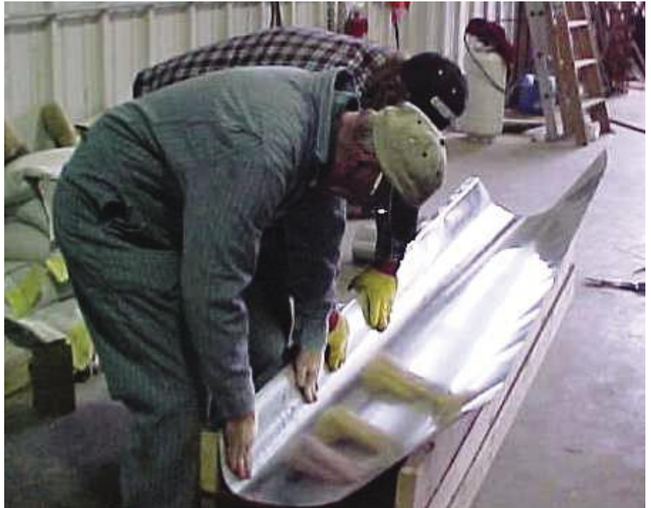
Building cattle guard base forms.
