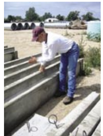
Gary Korell describing the installation of the bases.
