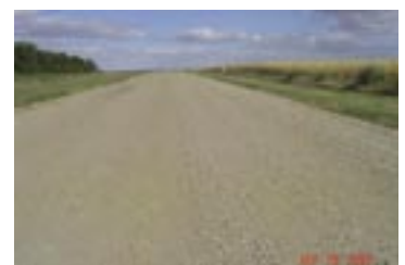
Outstanding performance of Douglas CO Rd #540-5 late in 2005 after a period of 41 days with no precipitation. Blade maintenance had been performed once during that period.
