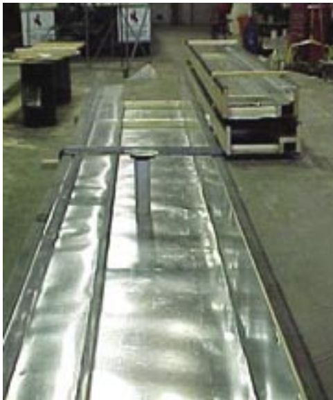
Forms with straps, keys, and PVC pipe to create handles.
