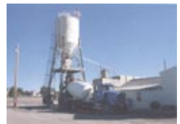
Sedgwick County Concrete Truck Loading
