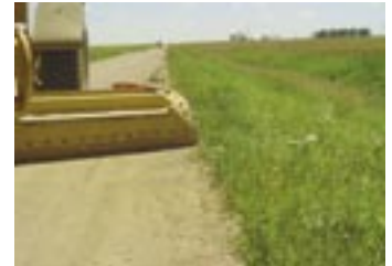
Rear view showing clean recovery of gravel at shoulder.
