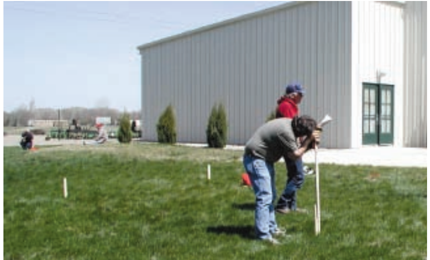
Off-set Grade Staking Crew
