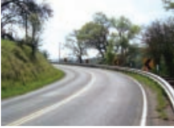
General view of county road system.
