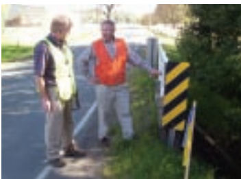
Ford and Grouchy viewing countywide standardized culvert treatment.
