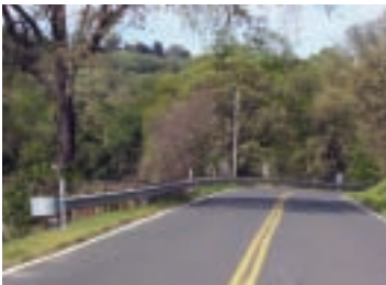
General view of county road system.
