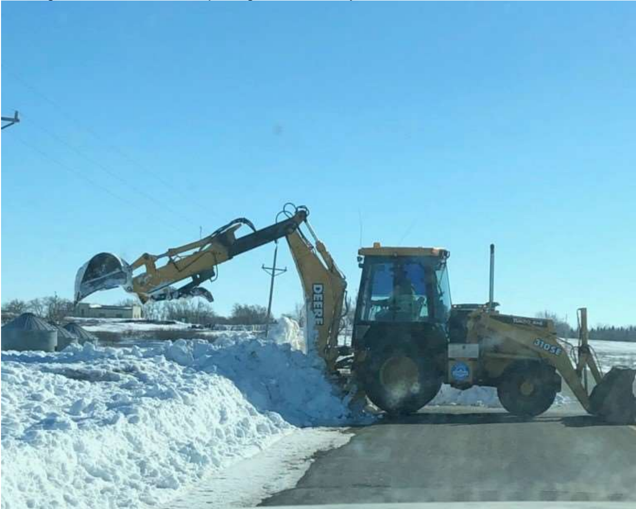
Busting snow in ditches and pulling onto roadway.
