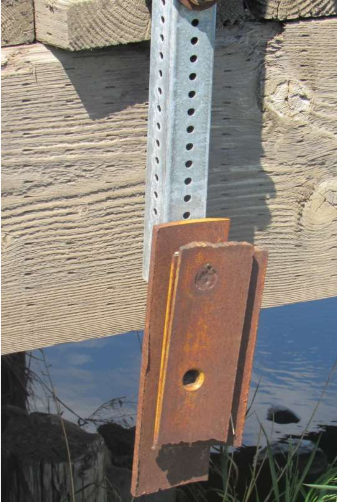
Counterweight – keeps sign in upright position.
