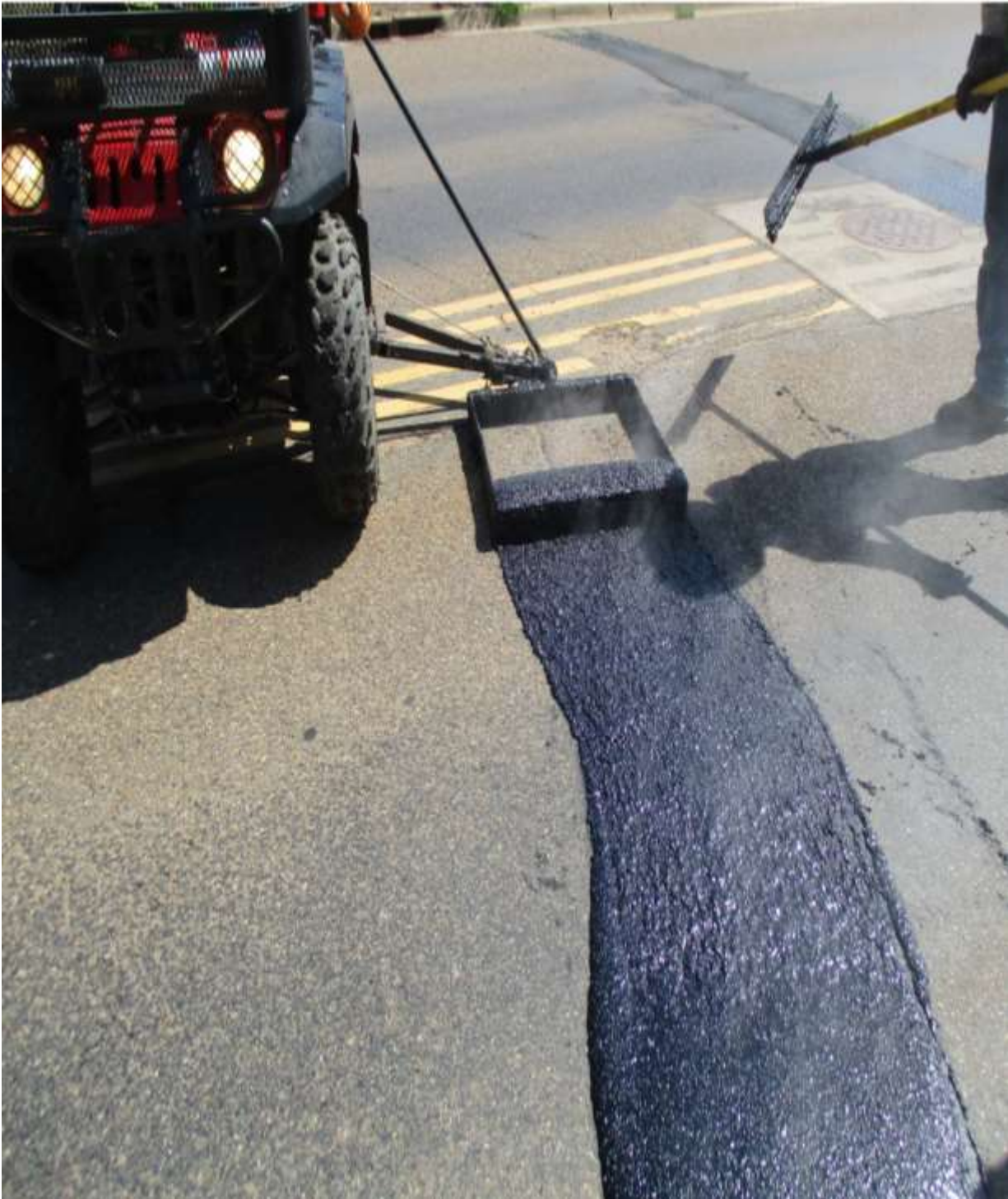
Crack Leveling Material Spreader (new method).
