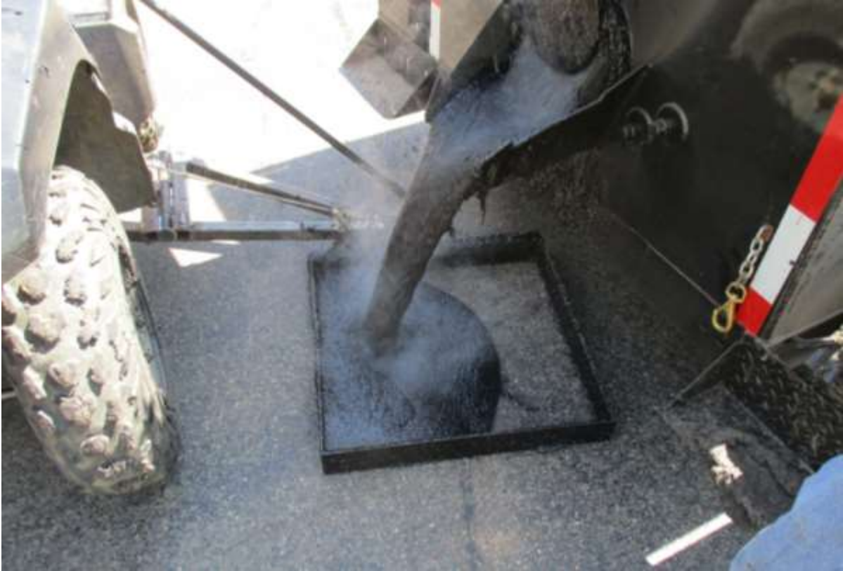
Filling box with mastic material.
