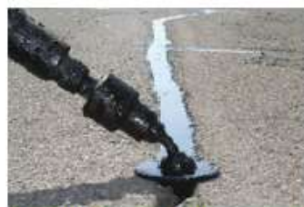
Routed crack being sealed
