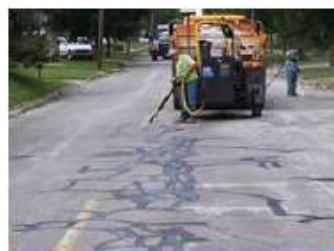
Crack sealing in the field
