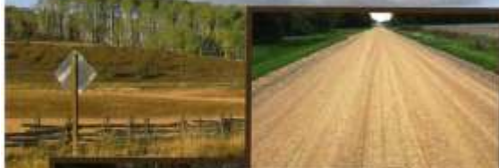
GOOD: Residential road, initial treatment 0.5 gal per sq yd. Same treatment Year 2. Gets 0.25 - 0.3 gal treatments in succeeding years. Treated annually 10 yrs. Performs very well.
