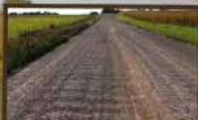
4/4 POOR: 10-7-13 After another 0.3 gal per was applied same season still not performing well. This is such poor surface material it won't go into a bound state no matter how you maintain it. There is no way the MgCl_2 can work even with 0.8 gal per sq yd applied in one year!
