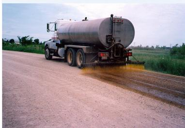
Dust control products could be sprayed by trucks used for applying asphalt products.
