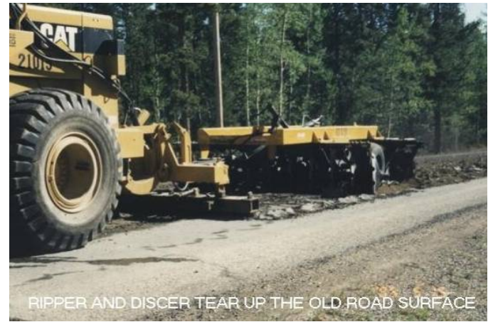
DISCER GRINDING UP THE OLD ROAD SURFACE
