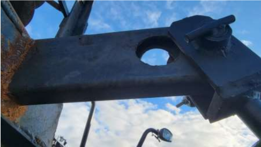
Tower for hydraulic cylinder
