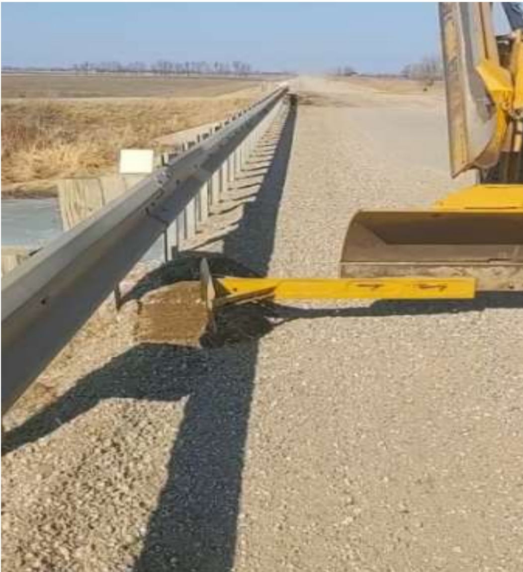
Pulling debris, gravel, vegetation that has accumulated between posts
