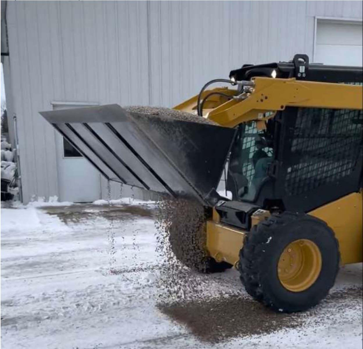
Chip Seal bucket spreader
