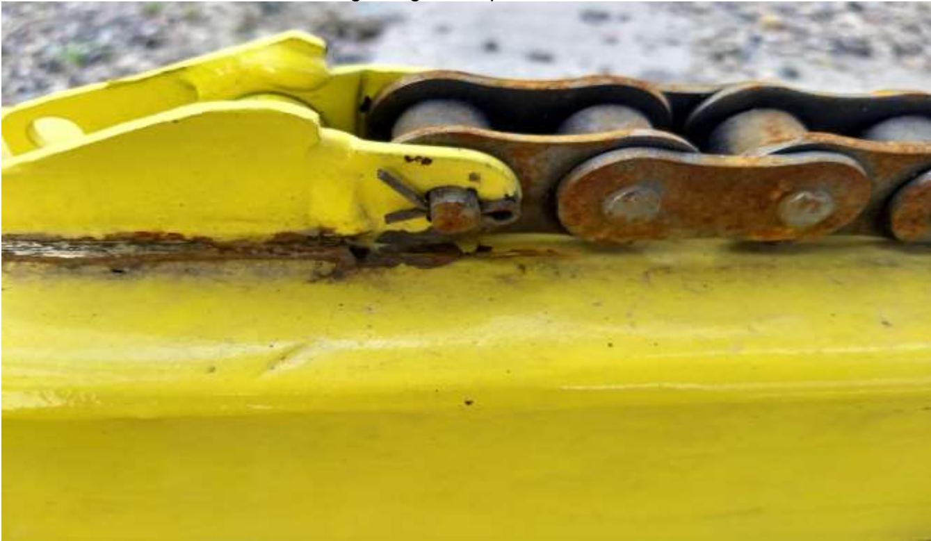
Link chain attached to 10-foot tubing using cotter pin and bolt.
