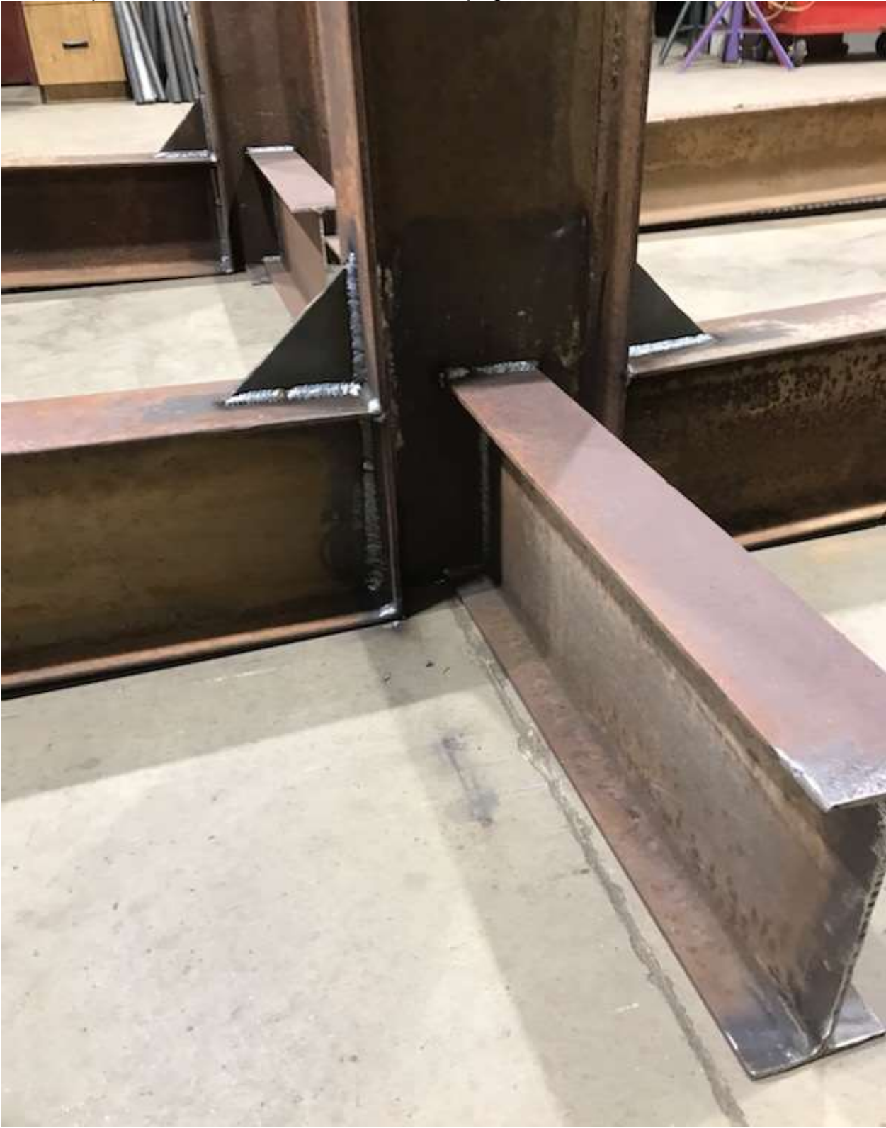
Gussets provide reinforcement for the 6-foot upright I-beam.
