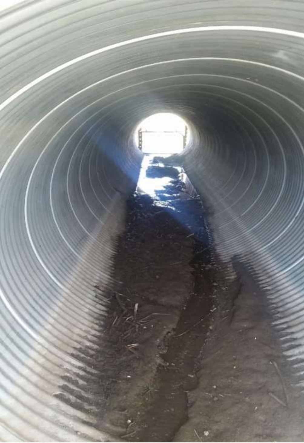
After: cleared culvert.
