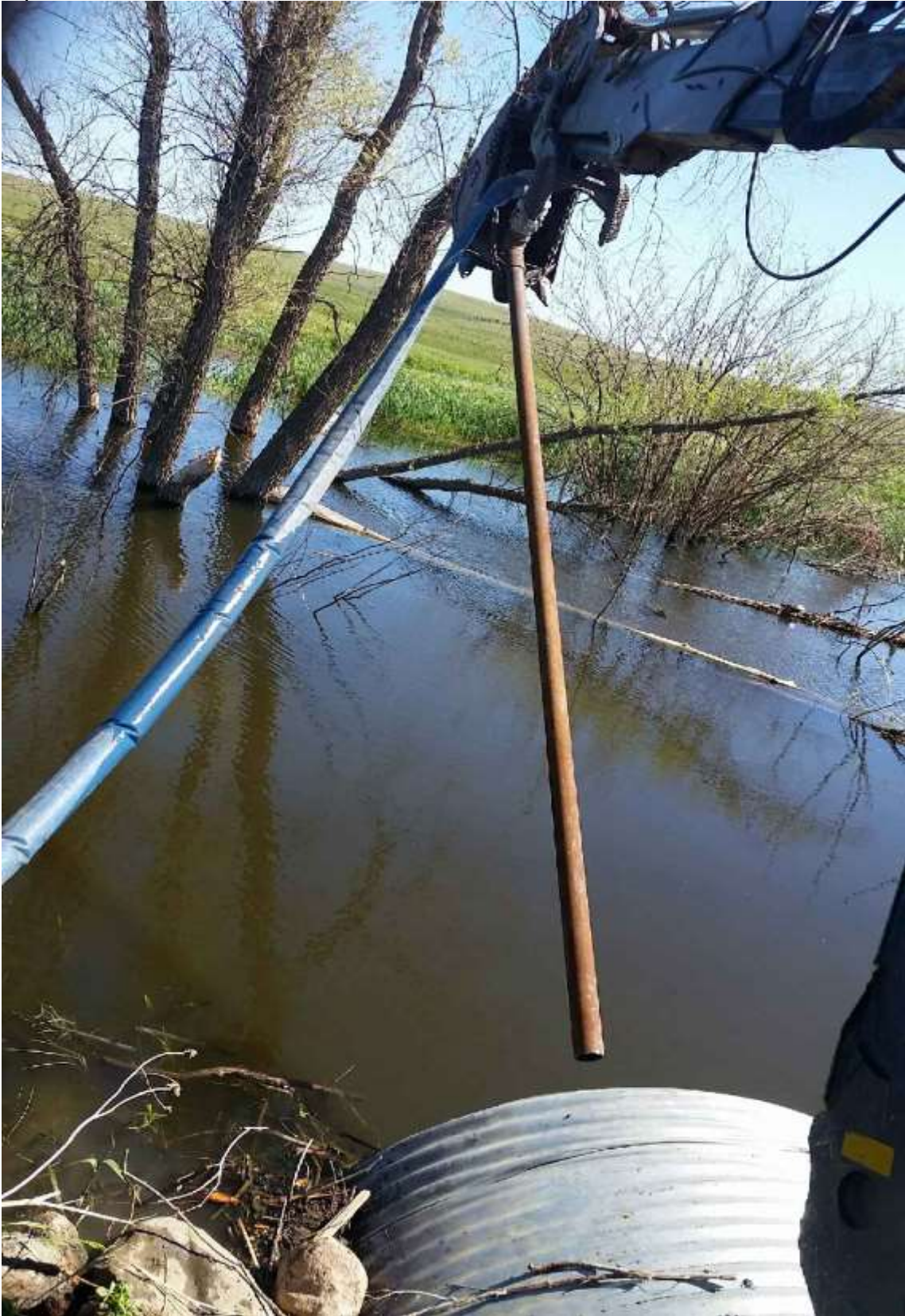
Pipe with water line attached to bucket.
