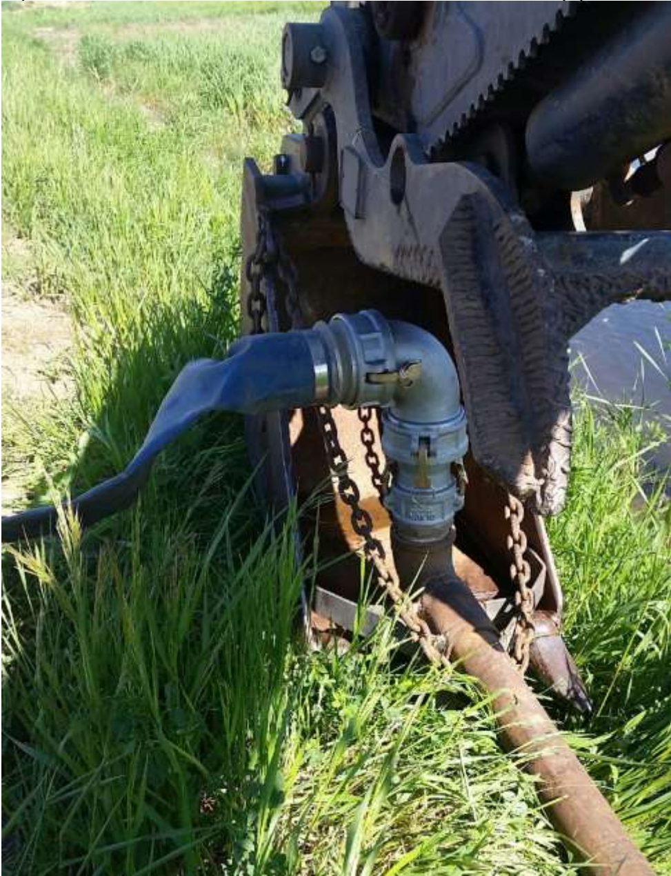
Pipe bolted and chained to bucket, water line attached to pipe.
