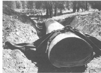
FIGURE 3 Filter bib placed around culvert pipe to prevent seepage and piping.
