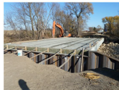
Sheet Pile Abutment
