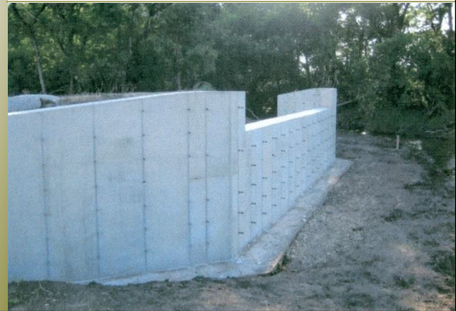
Completed Abutment
