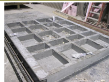
UHPC Waffle Bridge Deck Panels
