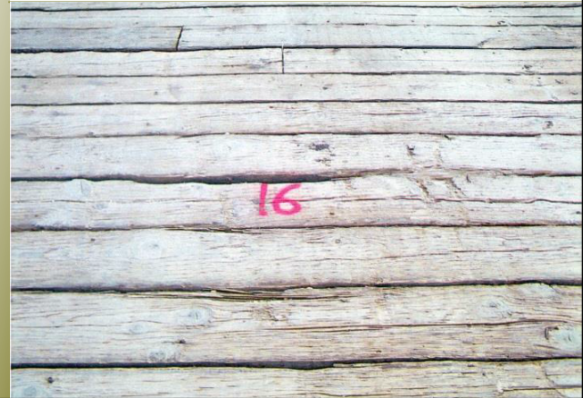
Original Bridge, Cracked Deck Plank
