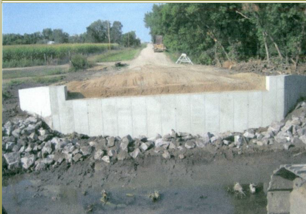
Completed Abutment with Riprap
