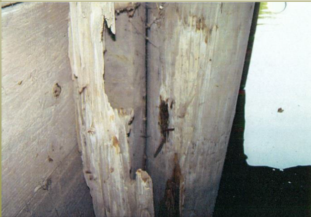
Original Structure Pile Rot, South Backwall
