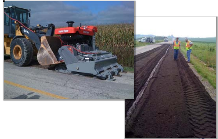
Small loader-mounted recycling machines have worked well on small projects
