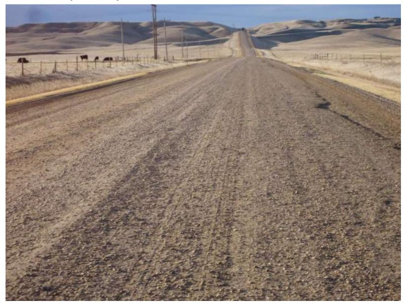
Some displacement of aggregate out of wheel paths
