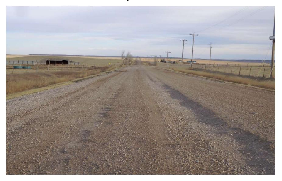
When crust breaks, the gravel erodes from surface quickly
