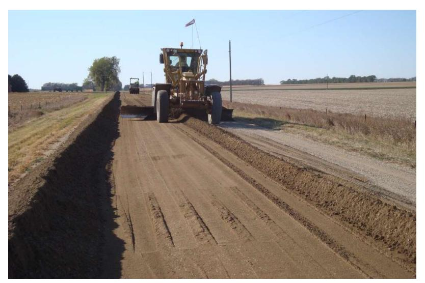
One of the biggest challenges was finding gravel that meets the modified SDDOT Specification: "Shall have minimum plasticity index (PI) of seven". (Even higher minimum was considered in project planning)
