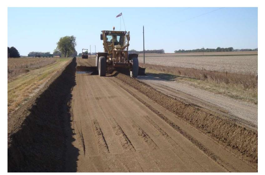
One of the biggest challenges was finding gravel that meets the modified SDDOT Specification: "<u>Shall have minimum plasticity</u> <u>index (PI) of seven</u>". (Even higher minimum was considered in project planning)
