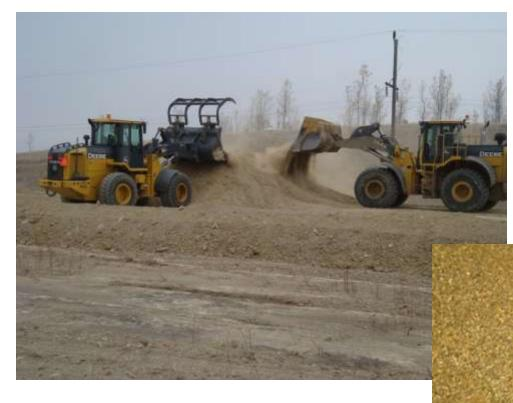
This was done on one section in Brookings Co and one section in Custer Co Is this the future? More blending or "manufacturing" to get high quality gravel – processing from a natural clay source here:
