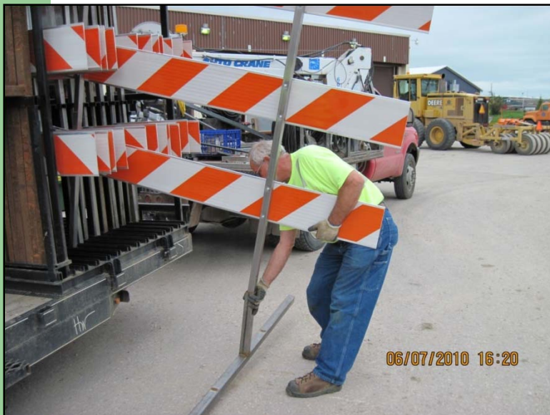
Barricade rack & aids in installing stand
