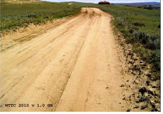
Washboards, potholes, loose aggregate and fear of isolated, substantial roughness reduces comfortable travel speeds.
