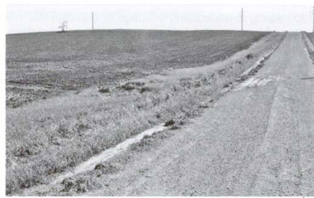
This road has a ditch badly filled with silt on the left and water overtopped in a recent storm
