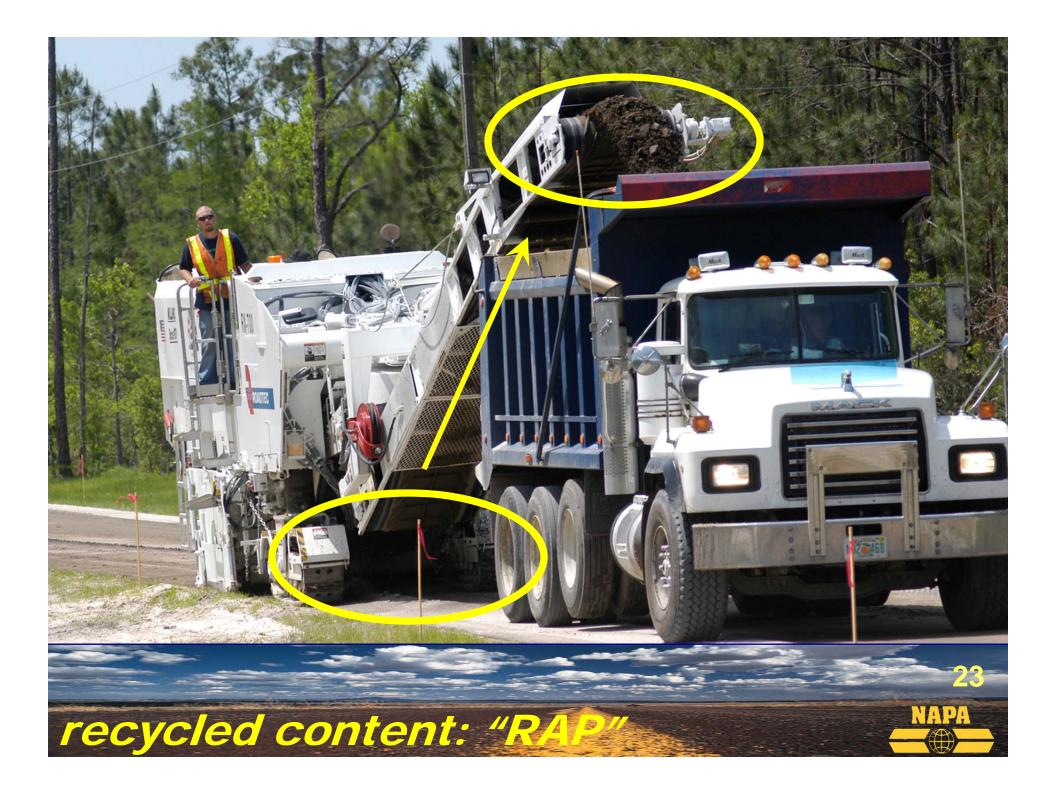
**Reclaimed Asphalt Pavement "RAP"** Removed and/or reprocessed pavement materials containing asphalt and aggregates Over 80 percent of the asphalt pavement, removed each year for widening and resurfacing, is re-used Represents close to 100 million tons / year RAP is the Nation's No. 1 recycled material in both total amount and percentage recycled
