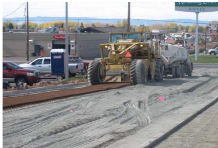
the curb and gutter. After the material was hauled back on to the site, ARS reclaimed the materials to ensure proper mixing and sizing of the old asphalt and base course. Normally, the asphalt and base course would be reclaimed in-place.
