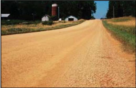
**Problem** Using straight cutting edges to cut out wash boarded roads disturbs more gravel than necessary.
