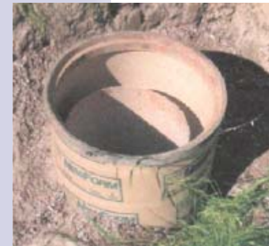
2008 Colorado State Winner Sonotube Drop Culverts
